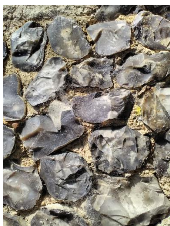
Knapped flint on the exterior of the south porch.
